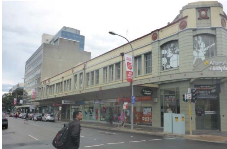
Figure 14: View west along Macquarie Street towards subject site, with immediate view heritage listed shop at 197 Church Street (Source: Urbis Heritage Impact Statement July 2015)
