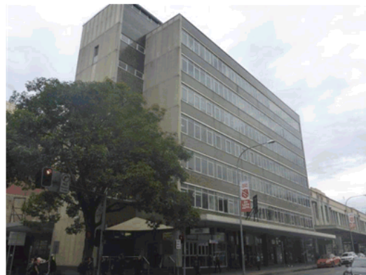
PICTURE 2 – THE SITE, AS VIEWED FROM THE INTERSECTION OF MACQUARIE STREET AND MARSDEN STREET
